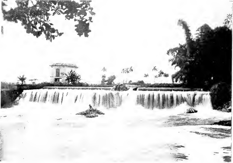
RESERVOIR OF THE OLD HAVANA AQUEDUCT.
